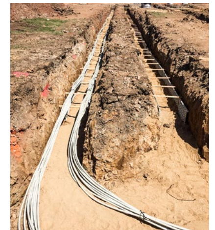
The flow pipes on the one side and the return flow pipes on the other: they are fixed above the collectors.
